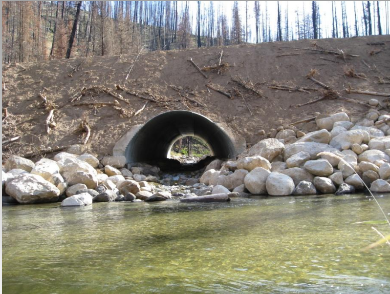
Goat Creek culvert after restoration; new aquatic organism passage (AOP), Payette NF
