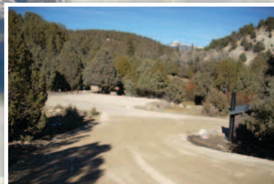
Second Crossing of Salina Creek
