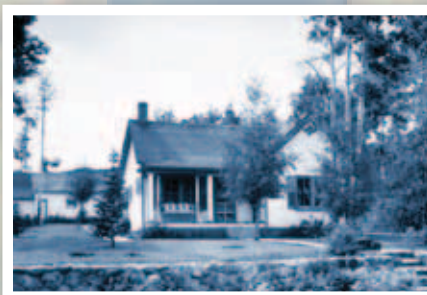
Gooseberry Guard Station
